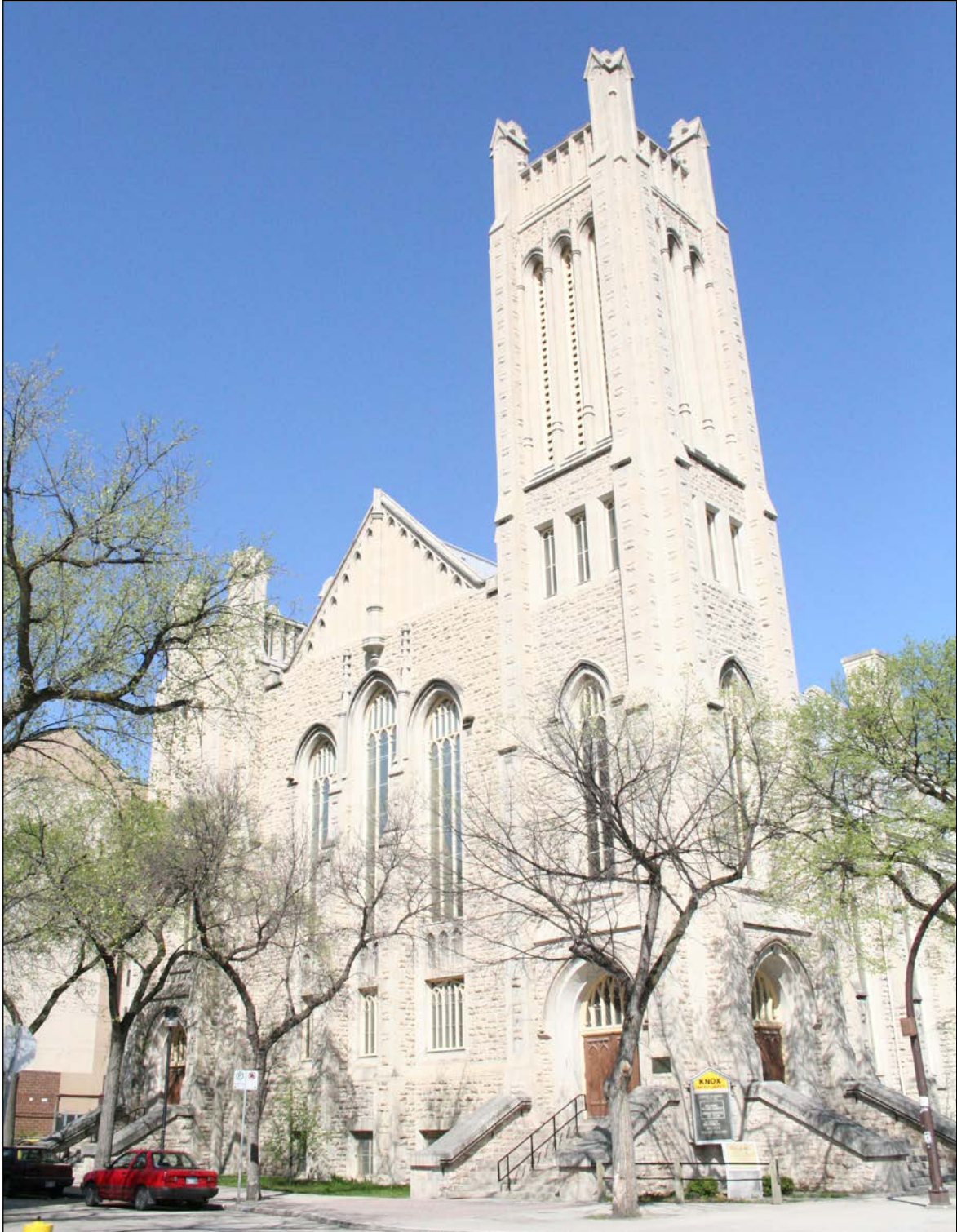
Plate 5 – Knox United Church, 400 Edmonton Street, 2007; built 1914-17, J.H.G. Russell, architect, James McDiarmid Company, contractor. ( M. Peterson, 2007. )
