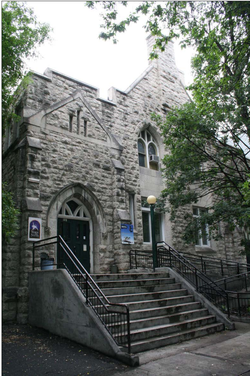
Plate 13 – Augustine United Church, 444 River Avenue, east side of Sunday School/Guild Hall Building, 2007. ( M. Peterson, 2007. )
