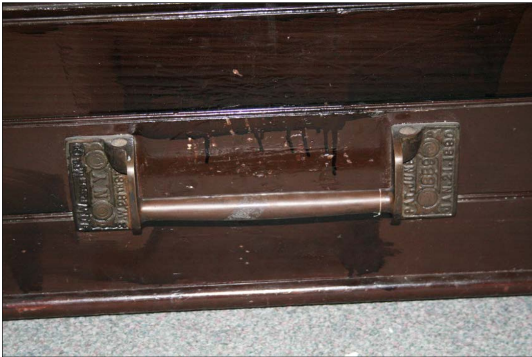
Plate 33 – Augustine United Church Sunday School/Guild Hall, original partition hardware, 2007. (M. Peterson, 2007.)
